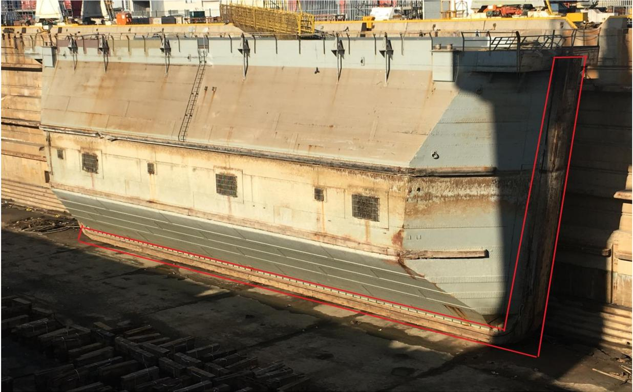
**Figure 2: SDD Floating Caisson Gate**
